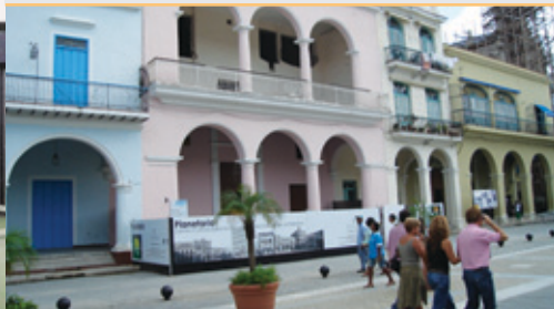
Figure 4 – Cultural Centre building under refurbishing
